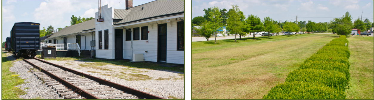
Exhibit 4-19: Existing Rail, Wooden Ties, Ballast, and Right-of-way without Track
