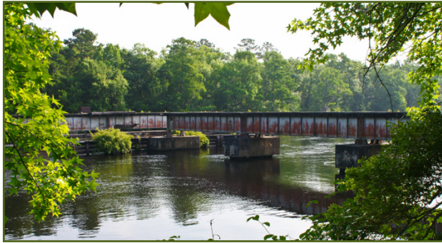
Exhibit 4-21: Northeast Cape Fear River Bridge and Deck
